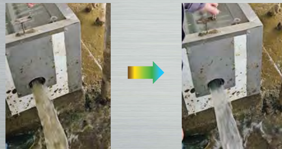
Step 3: Drain valve open, organic debris flushed from central channel.
